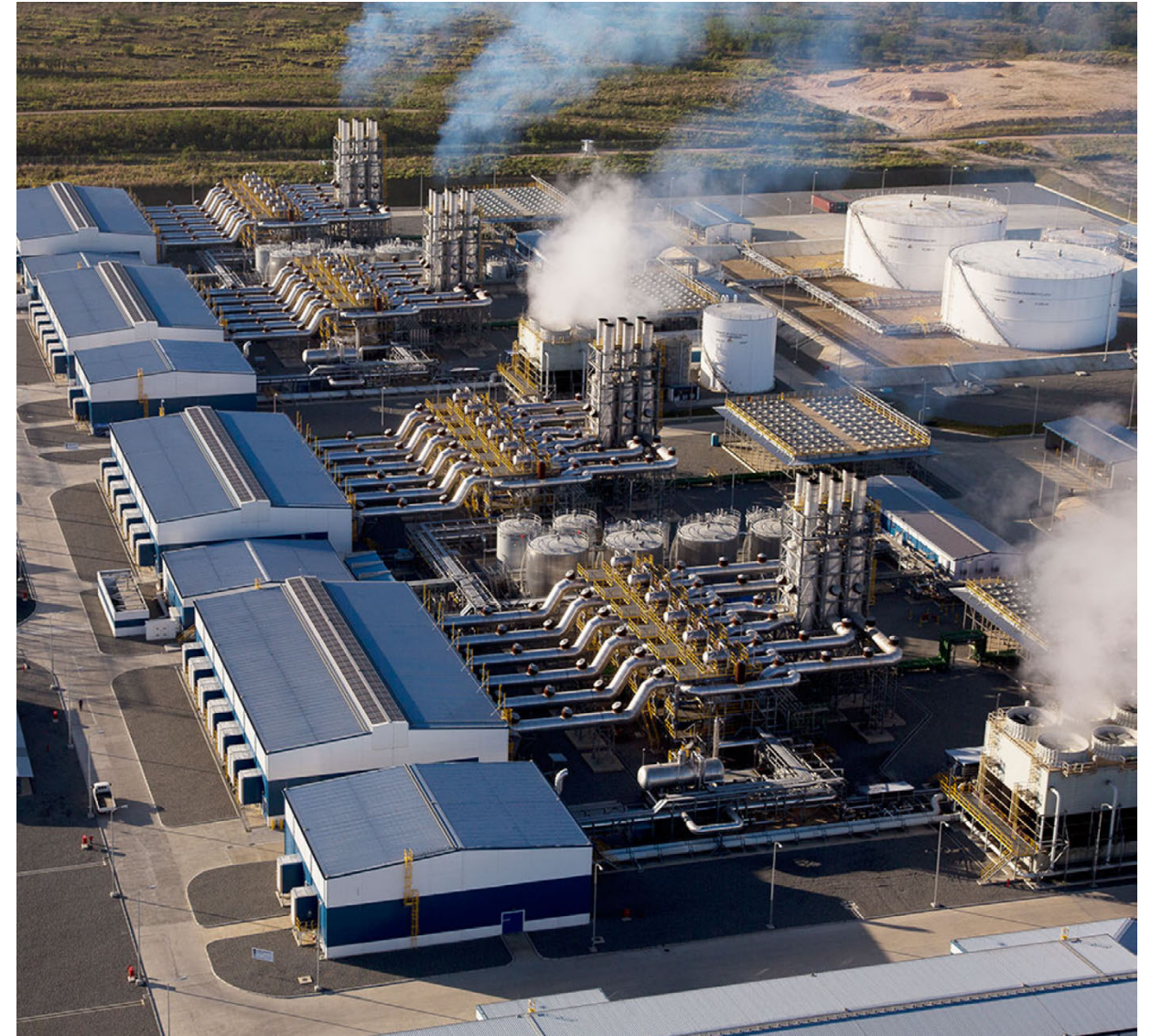
Quisqueya power plant, Dominican Republic
