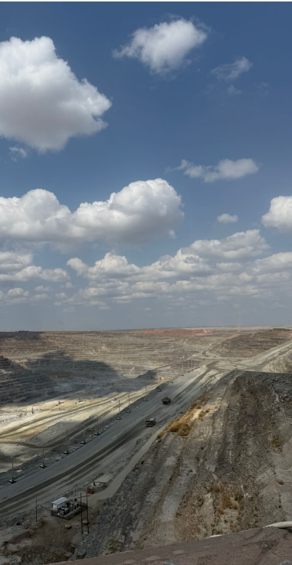
Electrified operations, Kansanshi site visit, 2025
